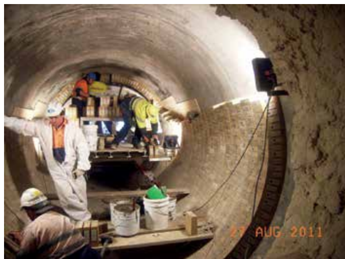
Figure 6: Installation of the Mag-Spinel brick on the insulation board below spring line
