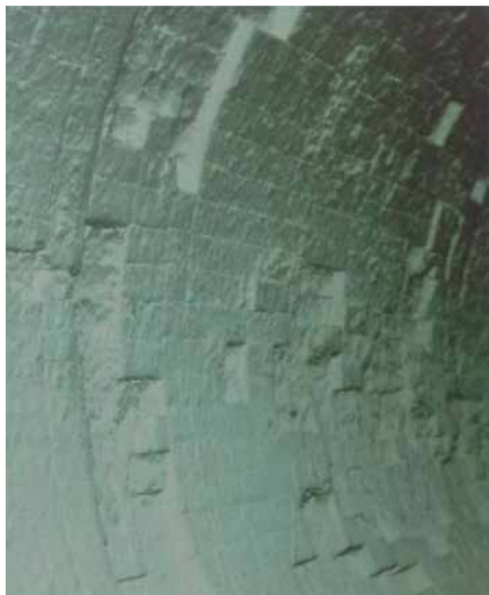
Figure 19: Spalling due to Ovality [9]
