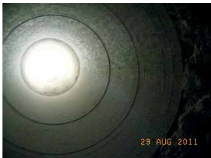
Figure 8: Installation of the brick on the insulation board completed
