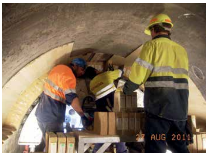
Figure 7: Installation of the insulation board above the spring line
