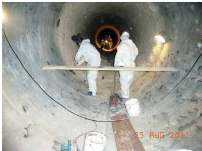
Figure 4: Picture inside the kiln showing removal of worn brick and shell preparation
