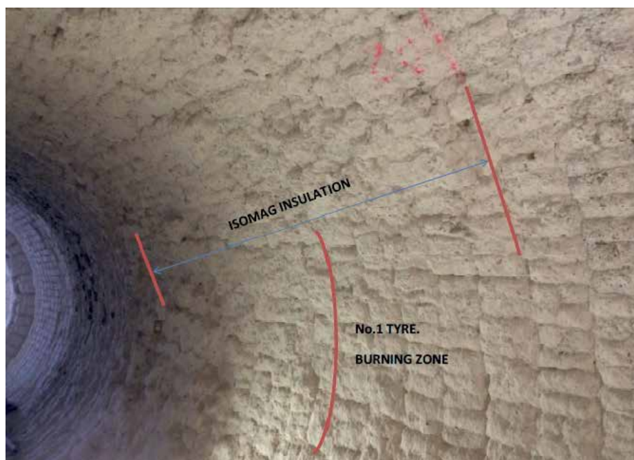
Figure 24: Wear Lining Brick – 28 months
