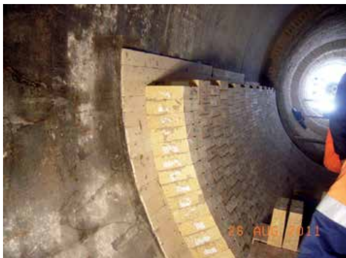
Figure 5: Installation of the insulation board across the shell bottom half
