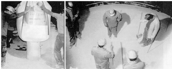
Electric Hearth Furnace Hearth: Use of dry vibratable basic material to construct or repair the hearth. Material is poured from a big bag, distributed manually into place and then consolidated using vibration skeds (think of installing block paving!)
