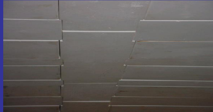
Sillimanite Tin Bath Roof
