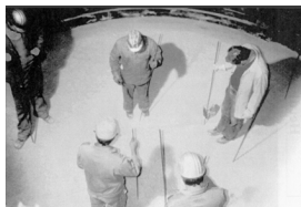
EAF Refractories: Installation of heath ramming
