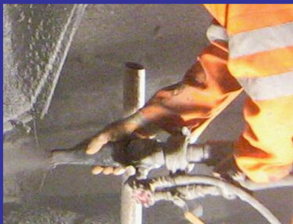
4. Special nozzle with air & accr
