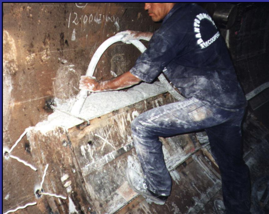
4. Apply high frequency poker
