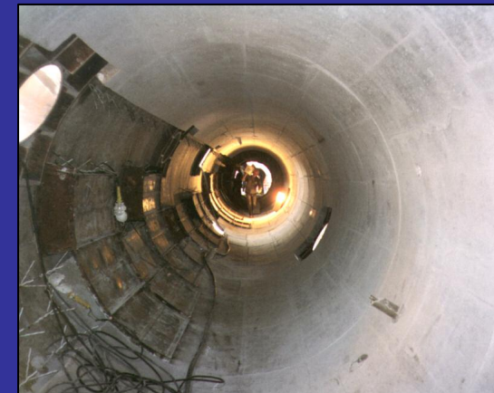
6. Partially completed lining
