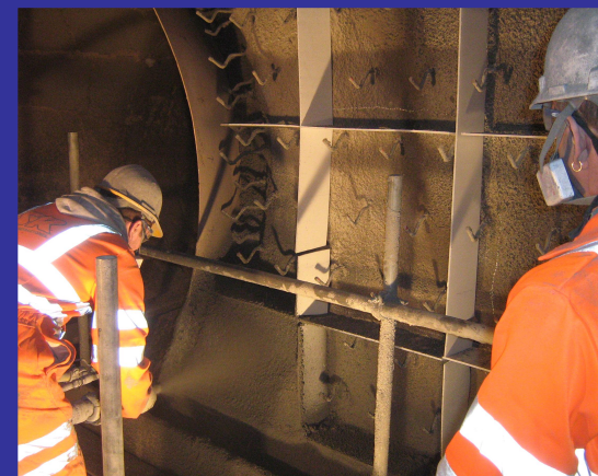
5. Applied in panels, quick setting (no slumping), clean environment
